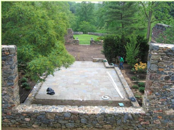
5. Preparation for sod installation
