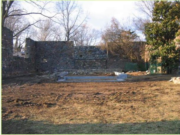
1. Initial site after patio base installed
