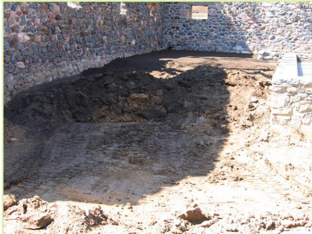
3. Compacted subsoil amended with Horticultural compost
